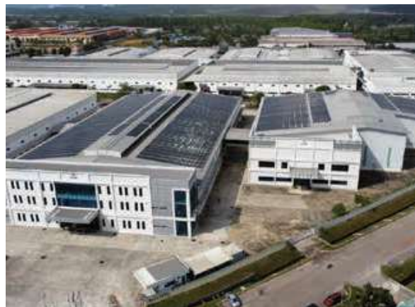
CA - Solar panels
